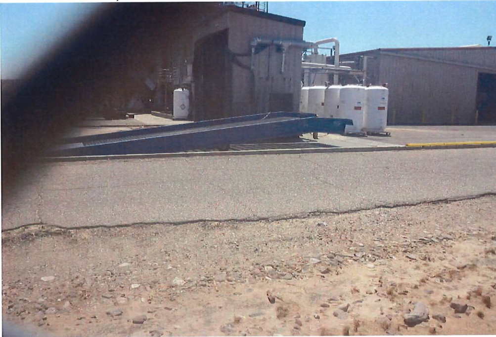
Photo 5: secondary containment around loading area
