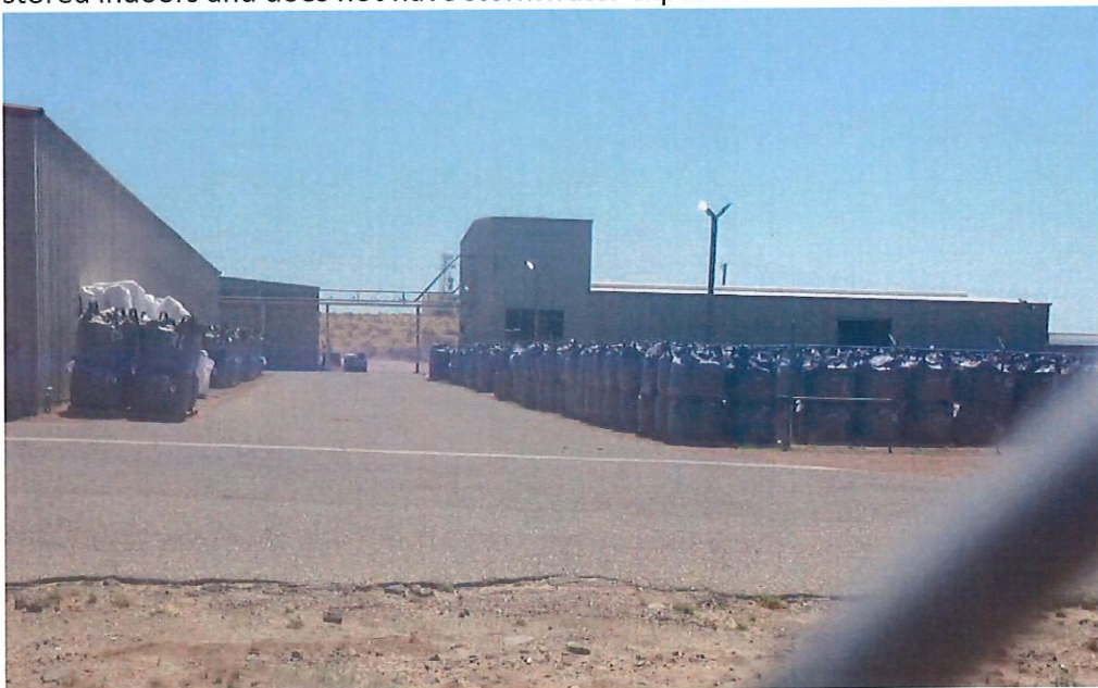
Photo 6: Outdoor Material Storage. All materials stored outdoors is clean re-activated carbon post processing and are contained in bags. All "spent" carbon received prior to re-activation is stored indoors and does not have stormwater exposure.
